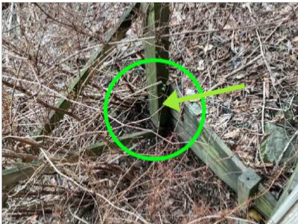
Earth mounted post with retaining wall at base
